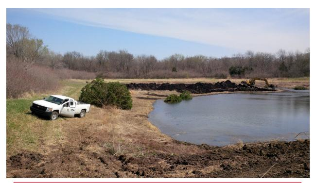
Above, USACE Park Rangers drag cedar trees to the waters edge to be installed for fish habitat as a contractor works in the excavator to dredge the pond and install a fishing pier. 2 of the largest ponds on Corps property were rehabilitated with this handshake agreement. Below, a contractor removes trees from a pond dam that is overgrown, damaged by muskrats and leaking water.
