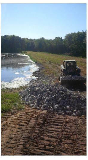
Left, USACE staff install 8 inch gabion rock along the waterline to protect the dams from muskrat damage.
