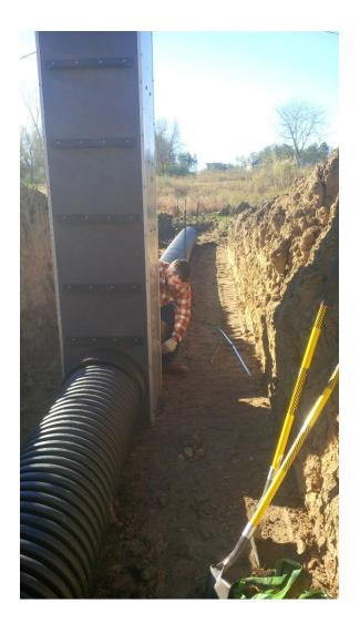
Left, Mitch Green, USACE maintenance employee attaches the inlet pipe to the water control structure at the wetland located at Public Access 31 on Smithville Lake. The existing structure had failed and no longer functioned to control the water levels. Below, USACE employees continue the backfill and compaction process to ensure a proper installation of the structure. 3 water control structures were replaced with this handshake agreement.
