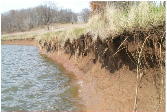
Above is a before picture of the heavily eroded shoreline at Sailboat Cove. The water level is at normal pool and continues to erode the base of the cut bank. Below, shows the placement of 6-14 inch rip rap along the shoreline of Sailboat Cove. The rock quarry's dump trucks back right up to the shoreline and dump 30 tons of rock at a time. These trucks weigh in at 80,000 pounds, so the ground conditions must be dry or frozen to get them off road.
